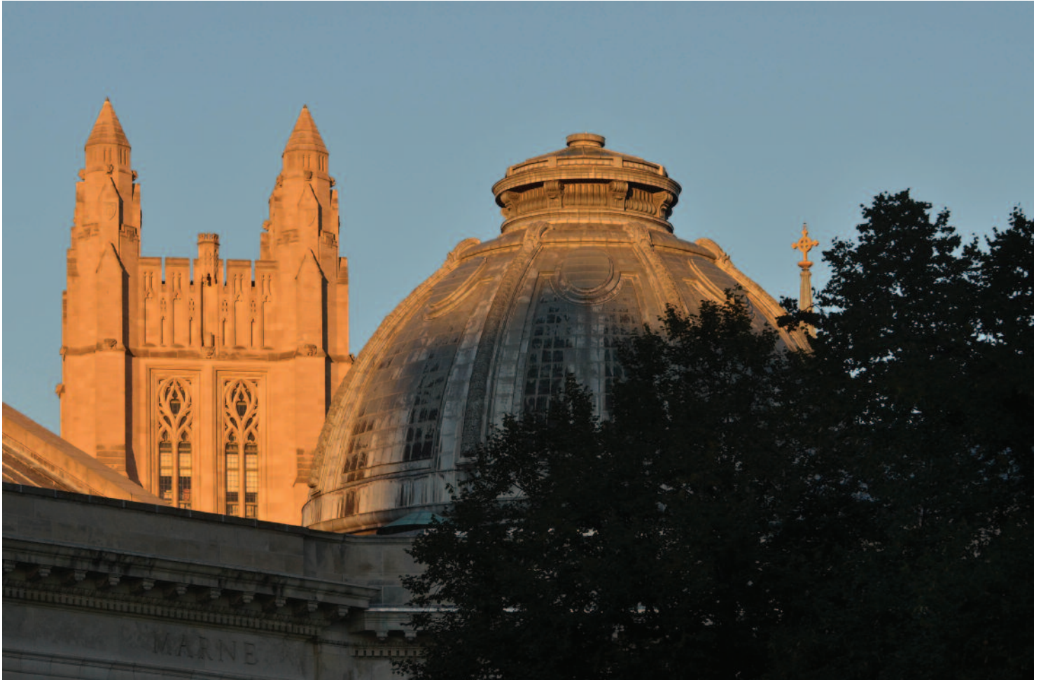
The rotunda above Memorial Hall, with Sterling Tower (part of Sheffield-Sterling-Strathcona Hall) at left.
