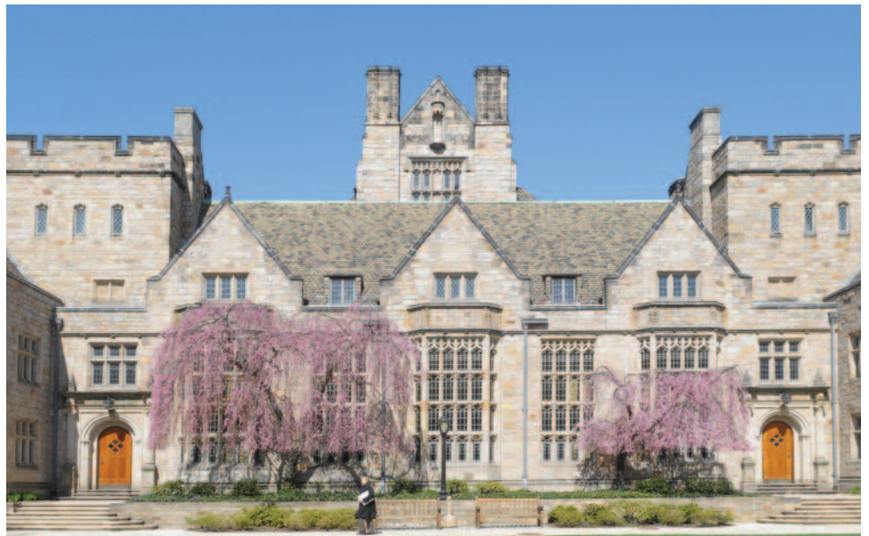
Exterior of Saybrook College dining hall.
