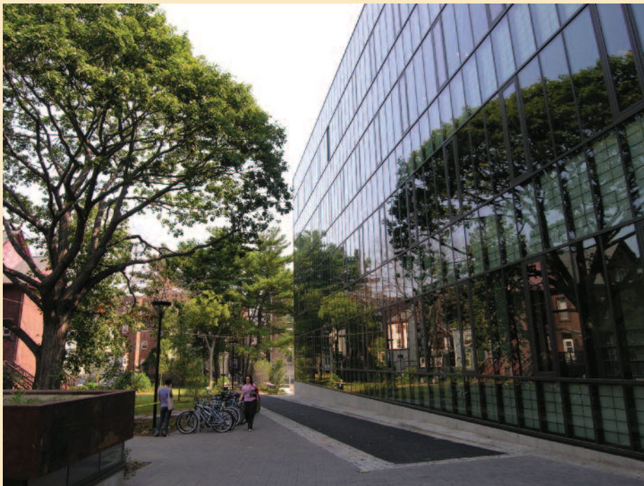
Green buildings are becoming part of the Yale landscape. The new three-story, 51,000 sq. ft. Sculpture Building houses undergraduate and graduate sculpture programs of the School of Art. The building's design features and construction process earned it a LEED Platinum rating from the U.S. Green Building Council. Kroon Hall (illustrated on page 9 in this report) has also received a LEED Platinum rating.
