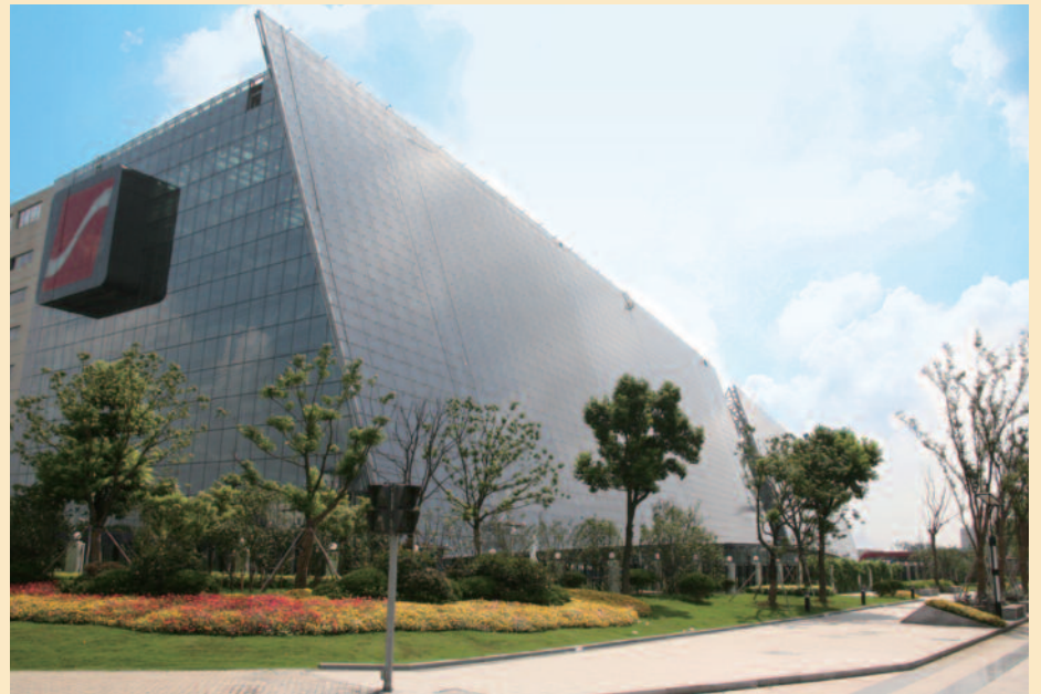
Suntech Headquarters in China.
