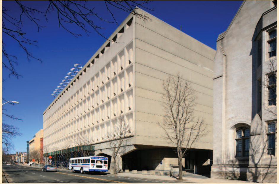
Two of Yale's sustainability efforts are illustrated in this view of Becton Center near the heart of the campus. Small wind turbines on the roof capture energy from wind currents traveling up the side of the building. Each turbine is 6.5 feet tall, weighs 60 pounds, and produces up to 1 kW of clean energy. The Yale Transit Shuttle seen in front of the building uses 20 percent biodiesel and 80 percent ultra low sulfur diesel. The Yale Shuttle provided almost 1 million rides to the Yale community in 2009.
