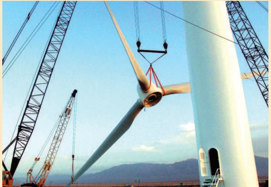
The development of Model HT40A/B blades (2.0 MW) was completed in 2007, and static and fatigue testing was concluded in May 2008. To date, 14 and 22 HT40A and HT40B turbine blades, respectively, have been manufactured and installed in wind farms in Inner Mongolia.
